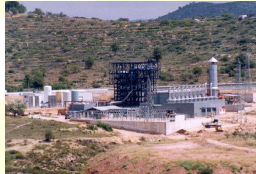
Poligas plant, Castellon (Spain) 25,000 t/y
